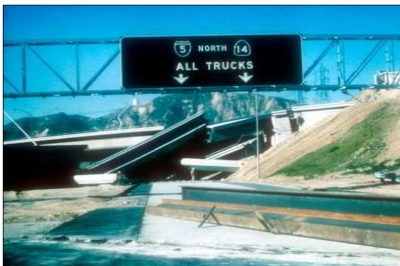
Earthquake damage to a bridge in USA, Route 5. (USGS, image in public domain)
