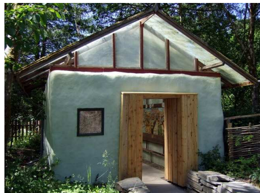
Straw bale building, Centre for Alternative Technology Machynlleth, Wales © ceridwen and licensed for reuse under this Creative Commons Licence
