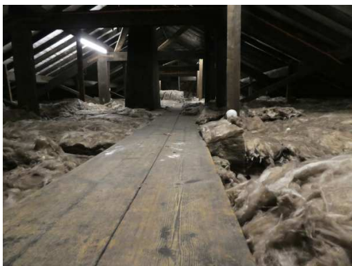
Fibreglass in the loft of a church Peter Kennett
