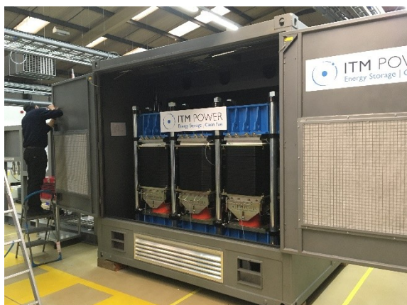
A 2MW electrolyser module under construction
