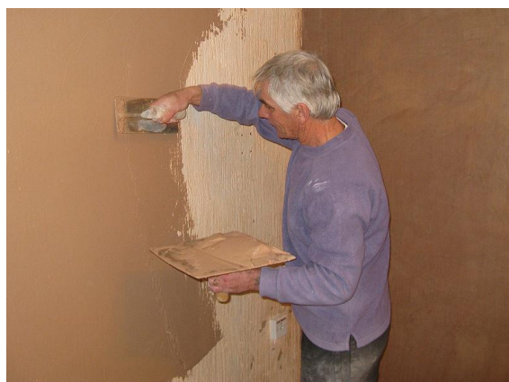
A craftsman plastering a wall (This work has been released into the public domain by its author, Arpingstone )
